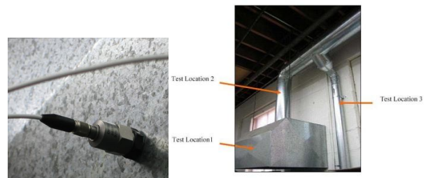
Fig. 6.1 Installation of accelerometer on duct
